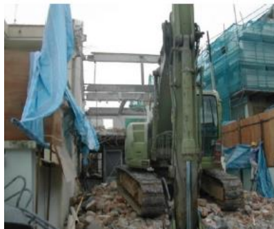
Demolition of a building
