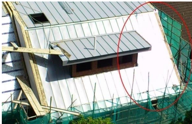
Diagram Ild.i: Shiny finishing which should be avoided when selecting material for your roof/façade
